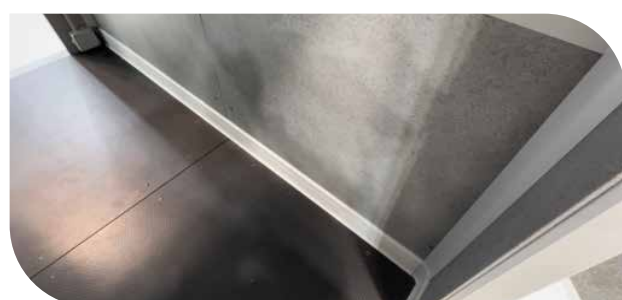
Interior PVC coating
